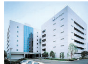
Kanagawa (Zama) <Sagamino System Laboratory (Registered Office)>
