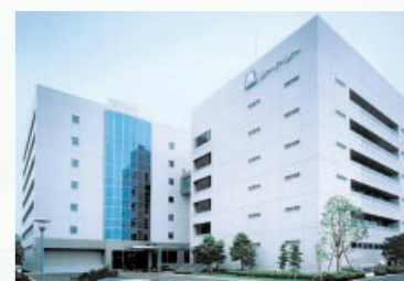
Kanagawa (Zama) <Sagamino System Laboratory (Registered Office)>
